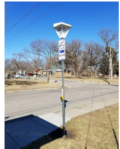
Pole Light, 10th St. at Highland Avenue
