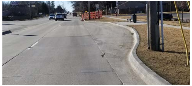
Pull-out Stop, 29th Street at Gage Boulevard
